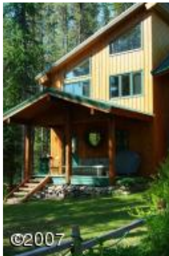
[2 of 15] EAST ENTRANCE
